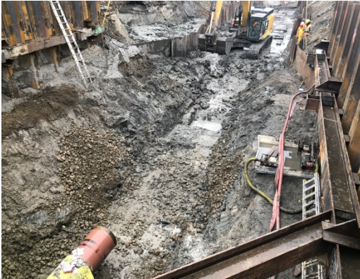
SF 8, oak creek crossing, most of the water is pumped out, pipe is visible.
