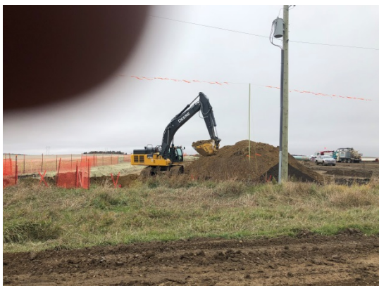
SF 28, photo facing east, excavator digging hole for where pipe will go under the road.
