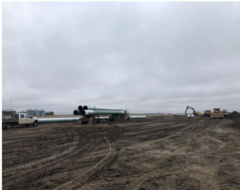
SF 14, photo facing east, stringing pipe taking place.
