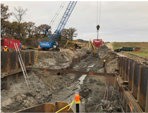
SF 8, photo facing west, oak creek crossing, excavator digging mud out of the trench, crews pumping water, machine tamping down steel support walls.
