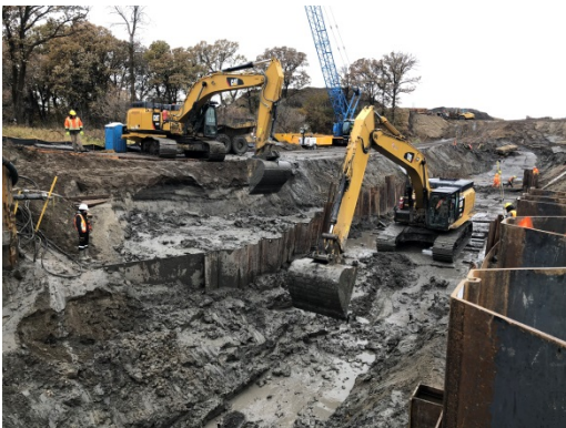
SF 8, oak creek crossing, two excavators and one rock truck working together to clear the mud out of the trench.
