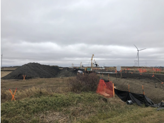
SF 47, photo facing west, pipe gang getting ready to move across the road.
