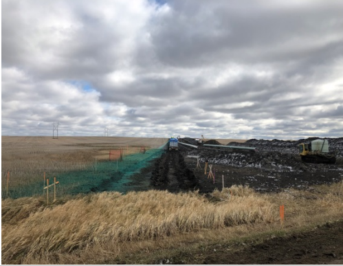
SF 43A, photo facing east, green mulch being sprayed.
