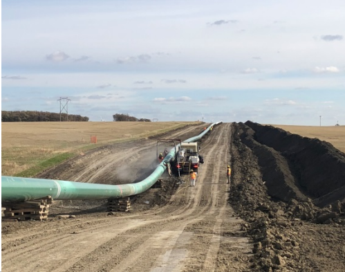
SF 44, photo facing east, coating crew sandblasting the welds on the pipe.
