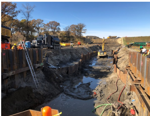
SF 8, oak creek crossing, photo facing west, not much has changed since yesterday, crews pumping water, hydrovac is on sight.
