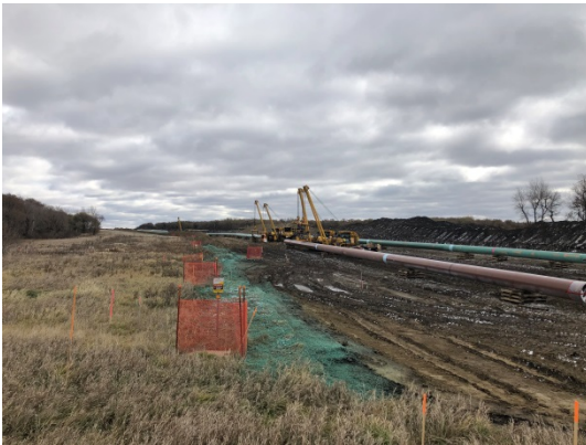
SF 38, photo facing south east, lowering in crew lowering the pipe into the trench.
