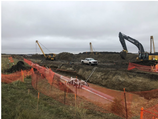
SF 22, photo facing south east, crews pumping water, lowering pipe in.
