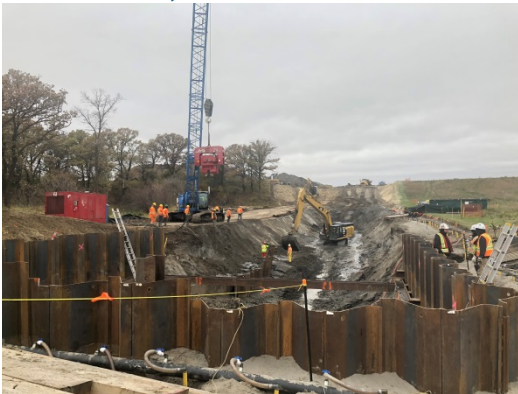
SF 8, photo facing west, oak creek crossing, crews pumping water out of pit, excavator moving mud out of pit.
