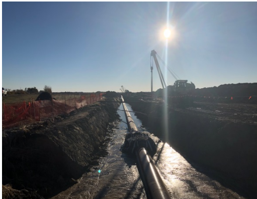
SF 22, photo facing south east, lowering in crew lowering in pipe, three side booms lowering in the pipe.
