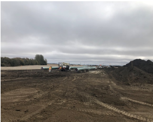
SF 38, photo facing east, coating crews coating the welds on the pipe.
