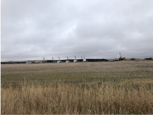
SF 43, photo facing south, pipe gang welding the pipe together.
