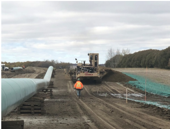
SF 39. photo facing west, trencher on sight trenching the ROW from west to east.
